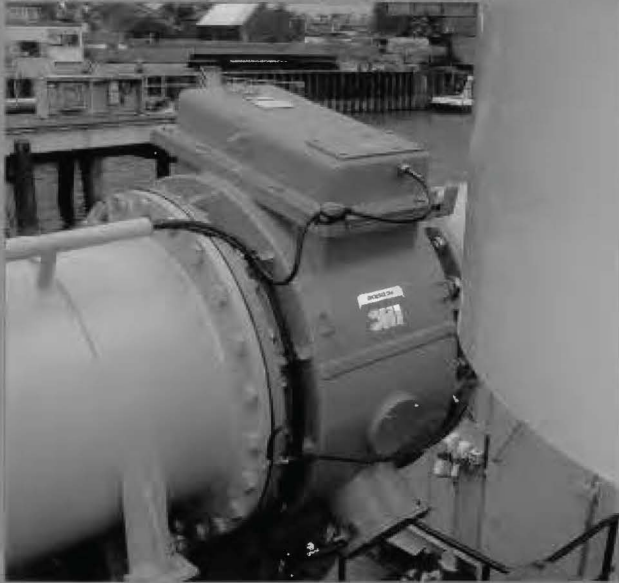
1.25 Integrated concentration and flowrate transmitter
