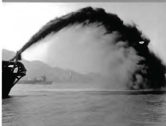
1.27 Dewatering is a natural part of the rainbowing process
