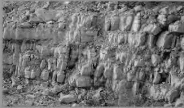
2.1 Soil in situ before excavation and...
